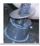
Inspect the whole louver including the base. Look for cracks and chips.
